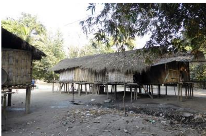
A Khot Kati, village Missing, Majuli)
