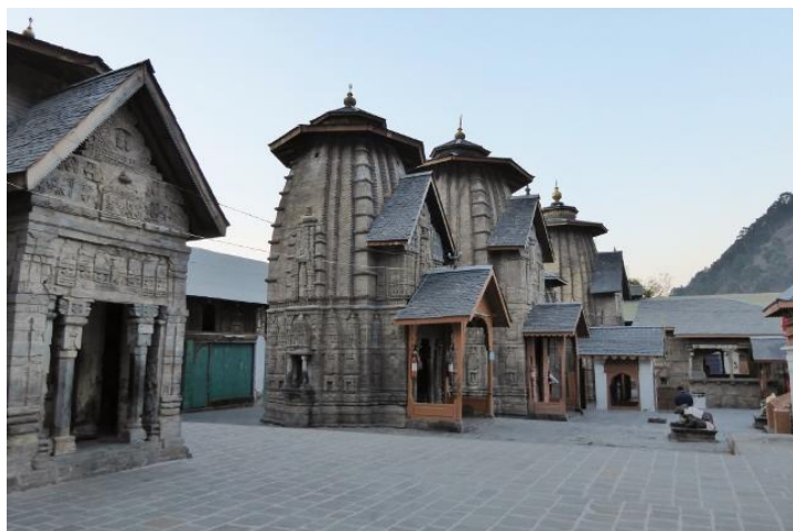
Alignements de shikharas, Lakshmi Narayan, Chamba
