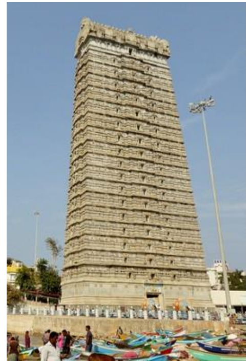
Gopuram (83 m), Murudeshwar
